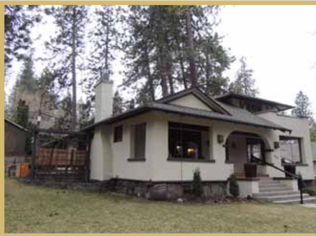
(Above) Two homes nominated to the Spokane Historic Register - the top one on Sumner Avenue and the lower one on West Shoshone.
