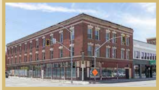
1907 Commercial Kehoe Building Olive Cooke 5002 North Market Street • Hillyard.
