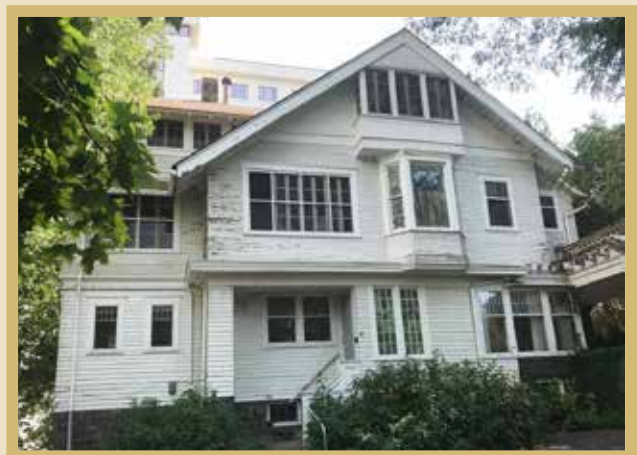
Recently Demolished Mary's Place by Providence Sacred Heart Medical Center.
